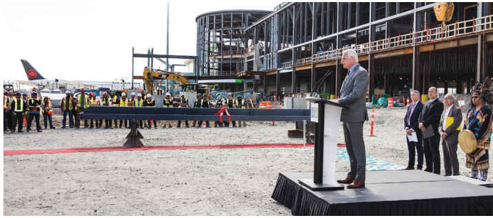
YVR CEO Craig Richmond speaks at a steel topping ceremony on June 4.
